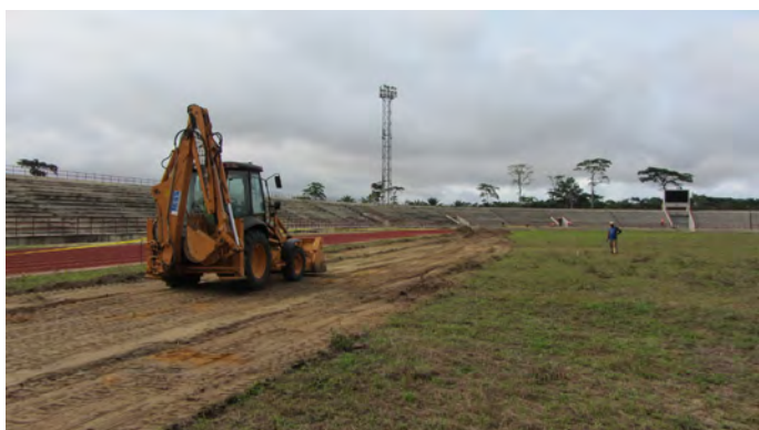
Figure 4: Vegetation and first soil layer removal.
