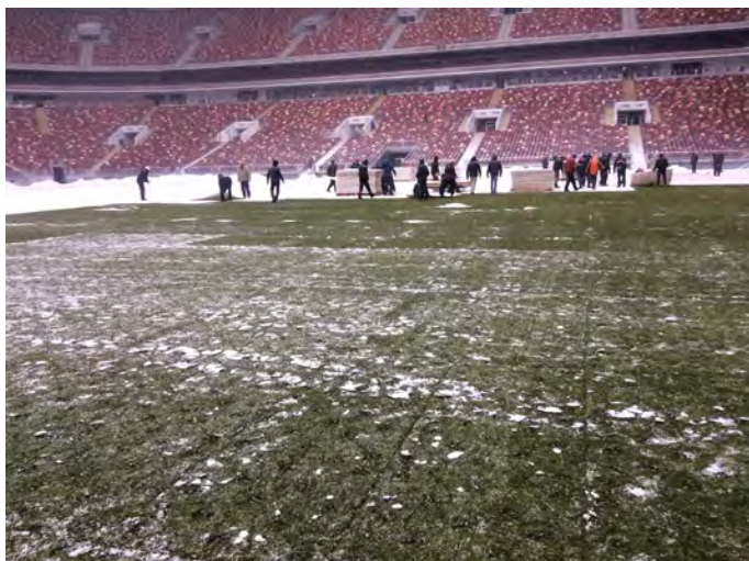
Removing snow off turf protection tiles that had been used to protect the Luzhniki Stadium pitch for an event in early March 2018, three months prior to the World Cup.
