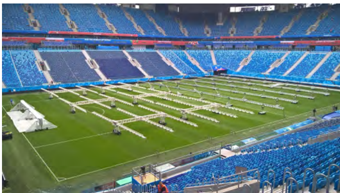
The extent of artificial lighting rigs used on the Krestovsky Stadium pitch in St Petersburg.
