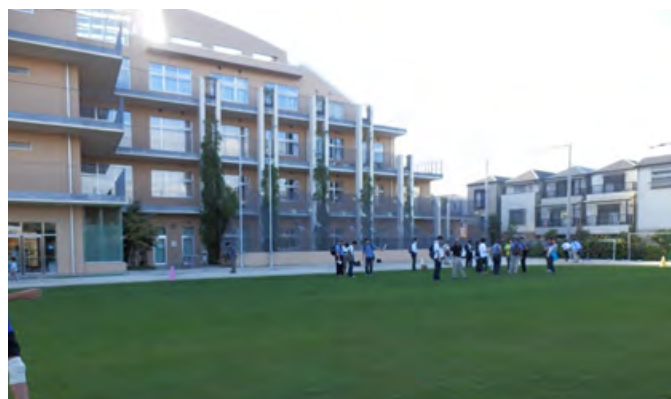
Amanuma Elementary School where the school building causes a turfgrass shading problem.
